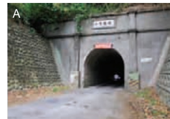
A | 小馬隧道除了兩端入口以鋼筋混凝土構築之外，其餘皆為人工開鑿的痕跡 | The Xiaoma Tunnel's entrance has been upgraded with steel reinforced concrete while the traces of hand tools have been retained in the rest of the tunnel.
